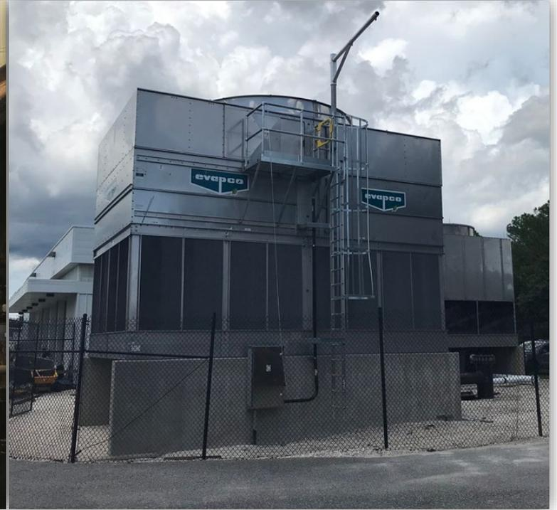
The expansion to the central chiller plant includes an additional chiller, and cooling tower in order to maintain compliance with the University's Campus Master Plan Policy to provide redundant cooling across campus. With the addition of the Applied Research Center, redundant cooling was taxed, so the additional chiller brings the University back to a state of  $n + 1$  redundancy.
